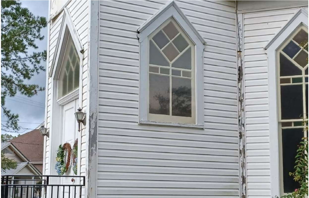
Existing fixtures to be replaced.
