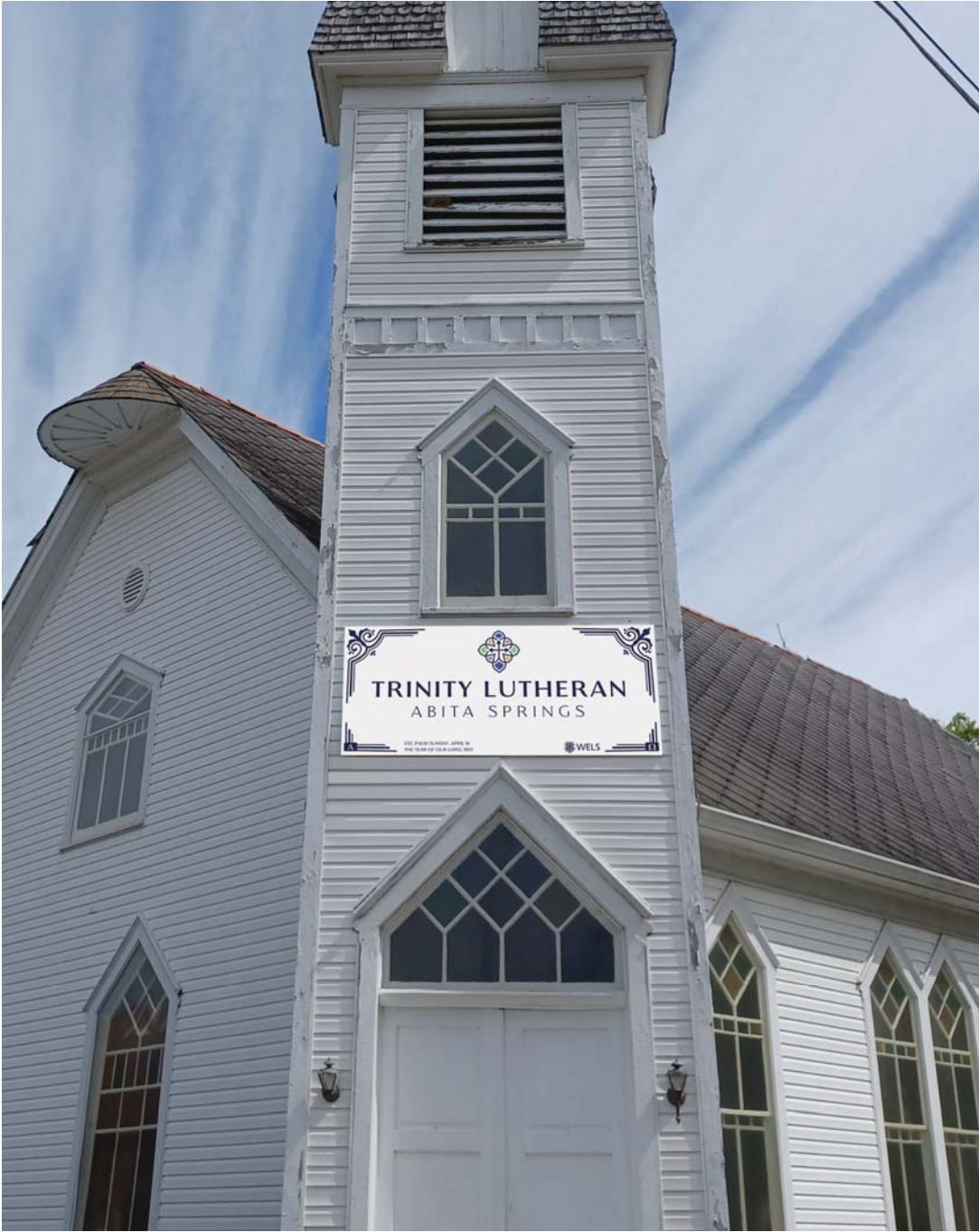
Detail View of New Signage
