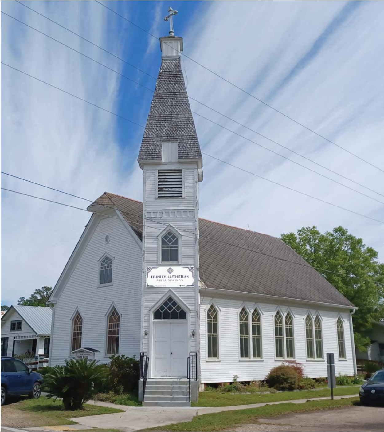
Street View of New Signage
