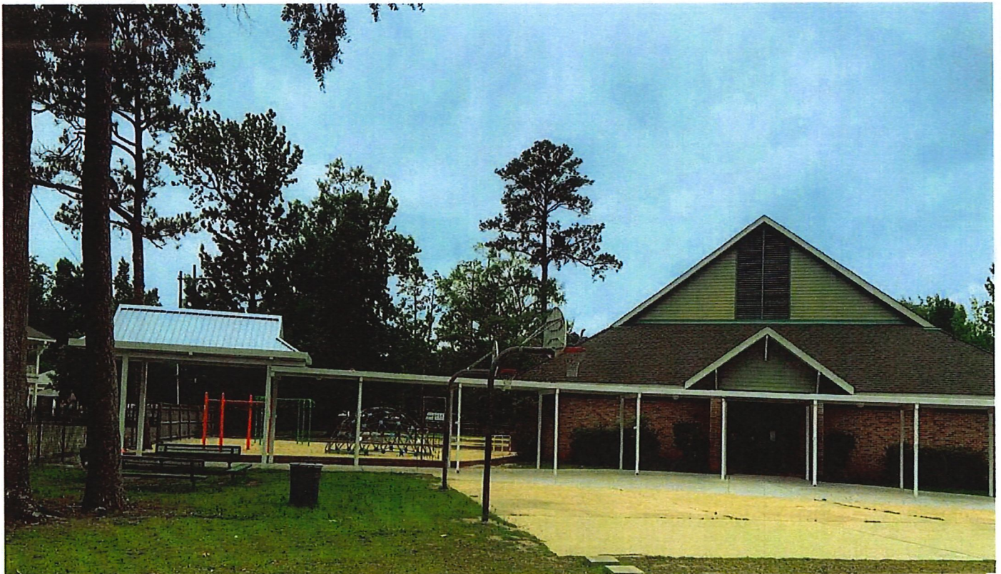
STREET VIEW FROM EXISTING FENCE
