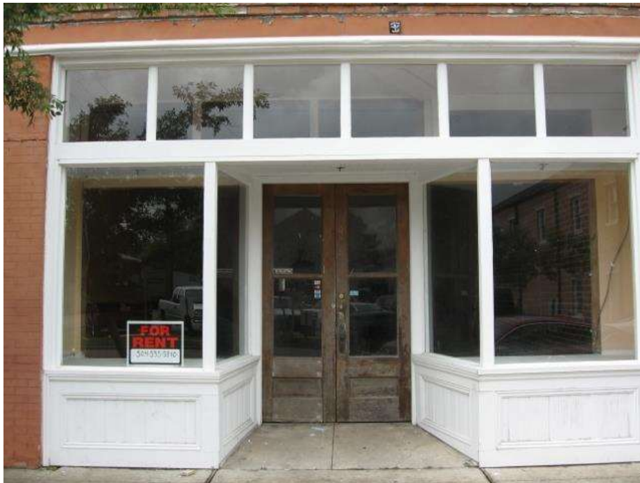
This new storefront was designed based on a traditional storefront plan of the turn of the 20th century. This storefront is similar to that recommended for Abita Springs as Façade Type A.
