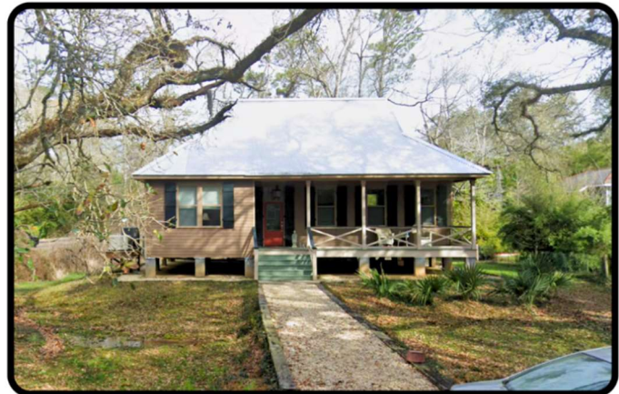
Example of compatible one-story infill construction at 22017 Second Street. The dwelling has a recessed porch, metal roof and pier foundation.
