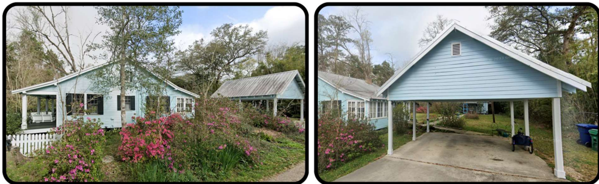
Appropriately designed carport at 71614 St. Mary Street.
