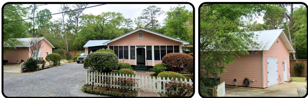
This garage at 72027 Laurel Street is an appropriate example of new construction and features a metal gable roof and hinged garage doors.
