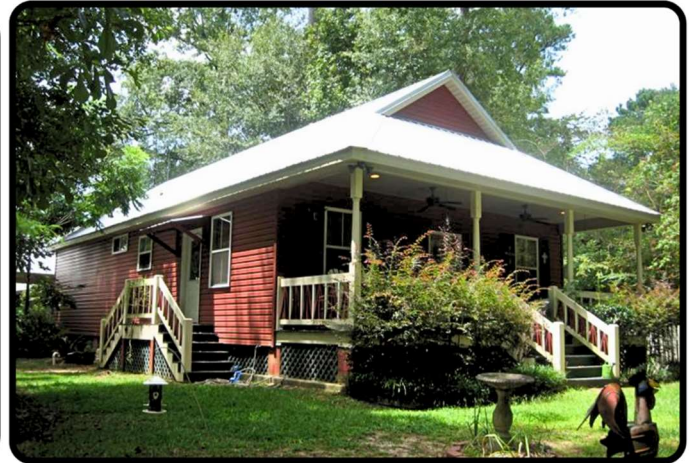
Example of compatible infill construction at 72059 Cypress St. Designed in a gable front plan, it has appropriately sized windows, a full-width porch, and a gable metal roof.
