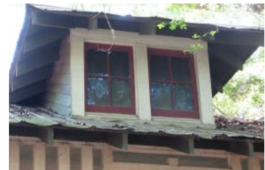
Roof features such as this hipped roof dormer at 71628 Leveson Street should not be removed or altered.
