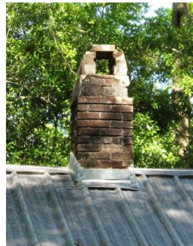
The brick chimney and its cap at 72125 Gum Street is an original feature and should be preserved.
