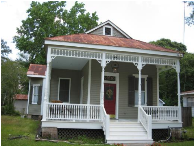
This Shotgun plan dwelling at 72110 Gum Street features detailed woodwork that is characteristic of the Folk Victorian style.
