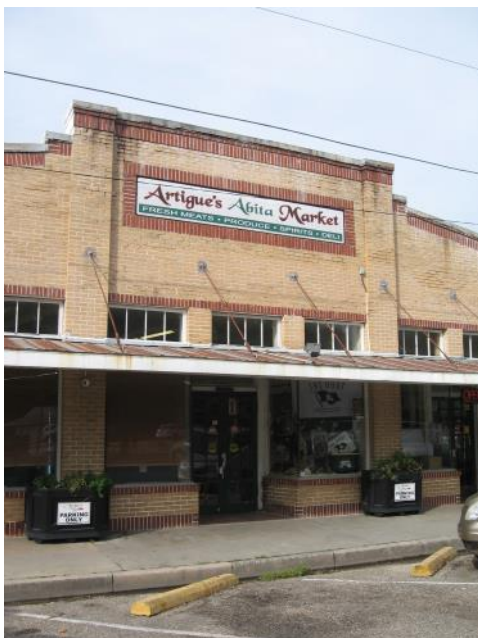
Retain historic awnings like the metal awning spanning the entire façade of the Abita Springs Market (22069 Highway 59).
