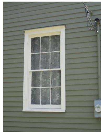
Original six-over-six, wood-sash window at 22222 Level Street.
