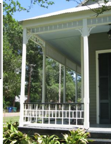
Porches are character-defining features in the historic district and original designs and features should be preserved and maintained (22222 Level Street).
