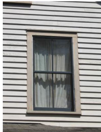
Example of an appropriate full-view storm window.
