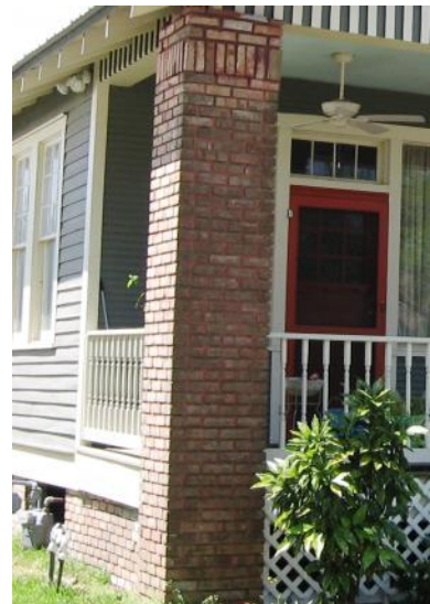
Brick is not a common wall surface in the district, but it is an important material for support features such as foundation and porch piers (22078 Main Street).
