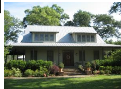
An appropriate infill design at 22145 Main Street
