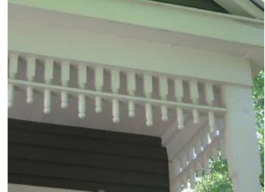
Trim such as this milled wood valance should not be removed or concealed (72170 Gum Street).
