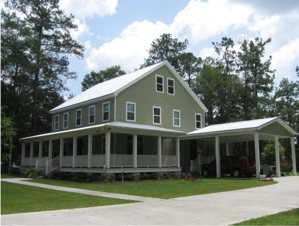
Example of compatible two-story infill construction at 22382 Level Street. The dwelling has a one-story wraparound porch, appropriately sized windows, and gable roof carport.
