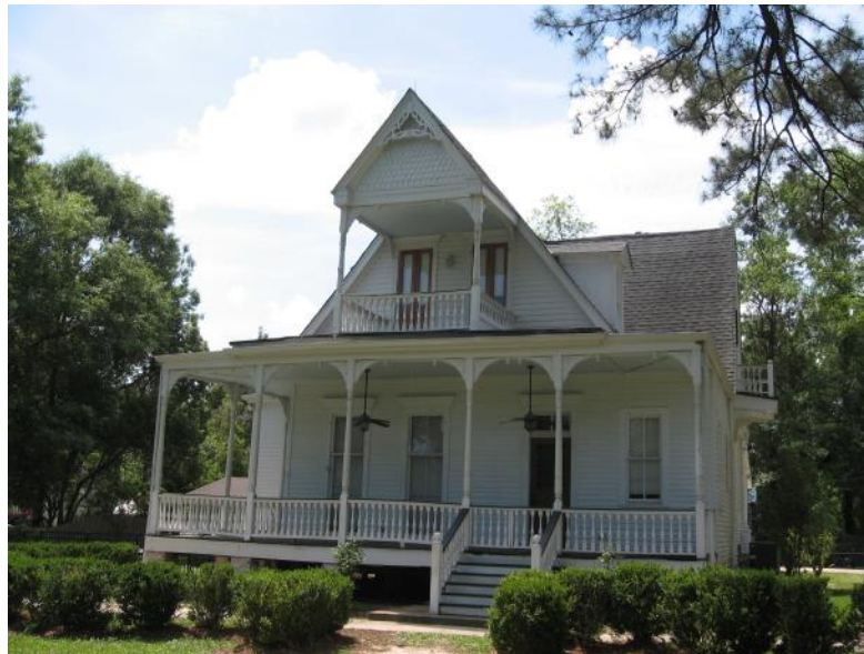
Example of the Queen Anne style at 71648 Maple Street which features a second story balcony and original milled porch columns.
