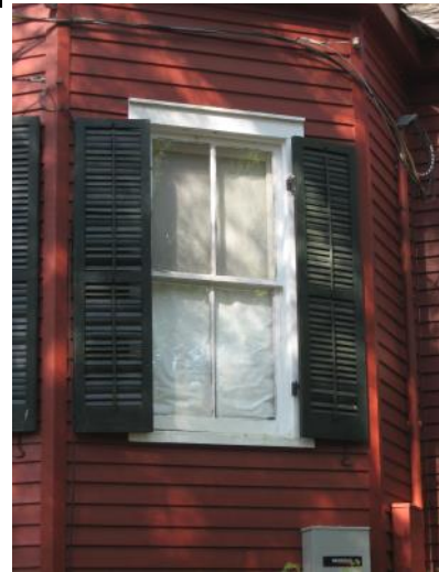
Original window shutters at 22205 Main Street.
