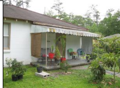
This metal awning dates from the mid-20th century at the house at 22324 Level Street.
