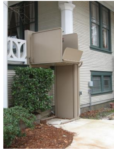
Chair lifts may be appropriate if sited on side or rear elevations, screened and reversible.
