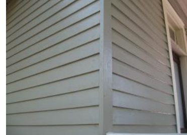
Retain and preserve original weatherboard siding as at 22179 Main Street.
