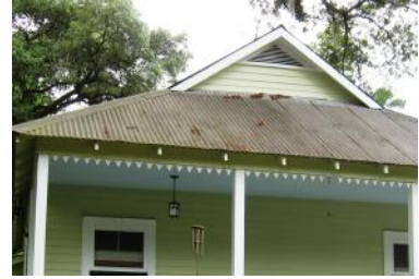
Many houses in the district have crimped metal roofs that contribute to the character of the building (71561 Hickory Street).
