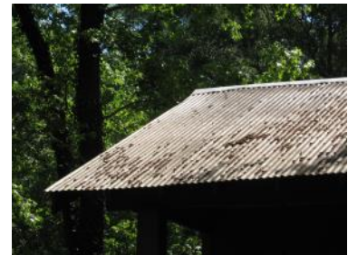
Close up of an appropriate crimped metal roof at 71620 Leveson Street.
