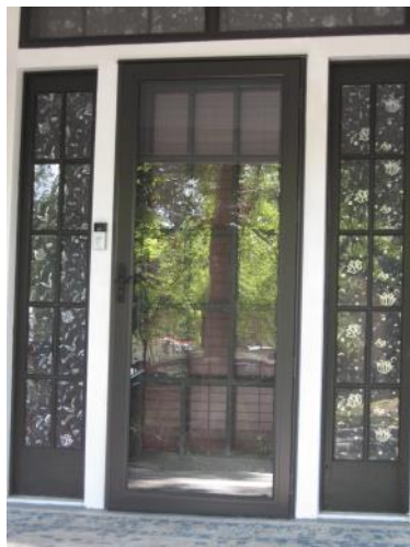
This full-view storm door allows the viewing of the original door behind it (72125 Gum Street).
