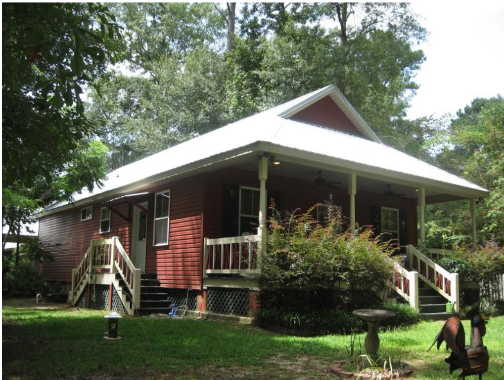
Example of compatible infill construction at 72059 Cypress Street. Designed in a gable front plan, it has appropriately sized windows, a full-width porch and a gable metal roof.
