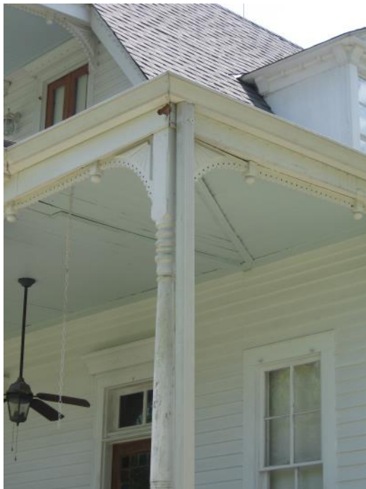
An appropriate gutter and downspout system at 71648 Maple Street.
