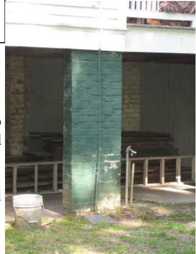
Brick pier foundation at 22166 Grover Street.
