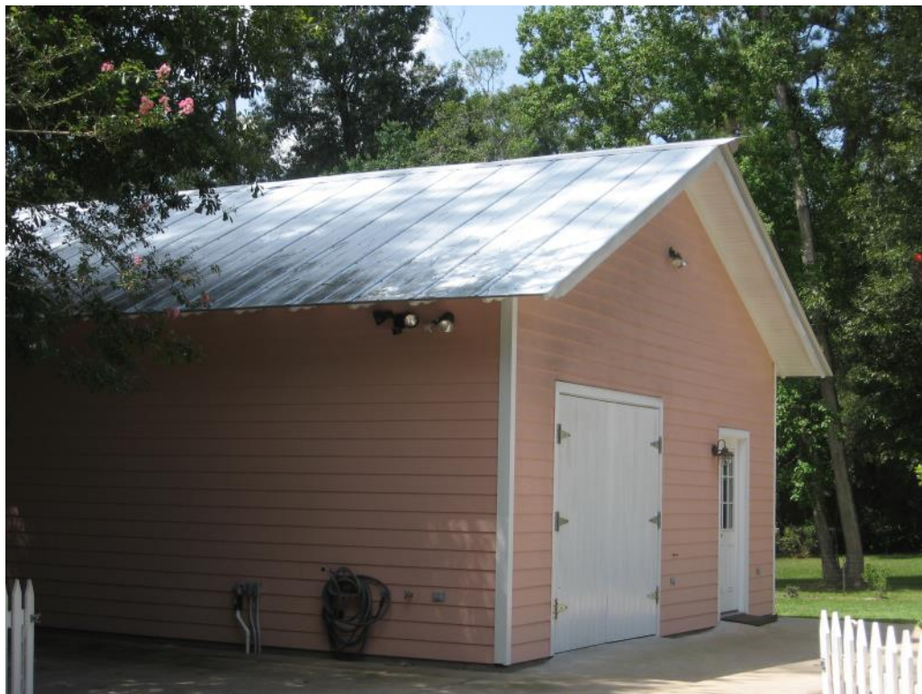
This garage at 72027 Laurel Street is an appropriate example of new construction and features a metal gable roof and hinged garage doors.
