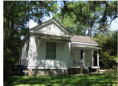
A gabled ell dwelling at 11613 Keller Street.
