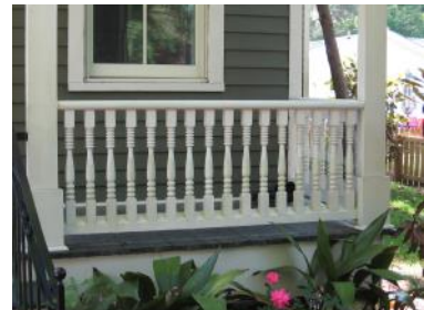
Original porch railing at 72170 Gum Street.
