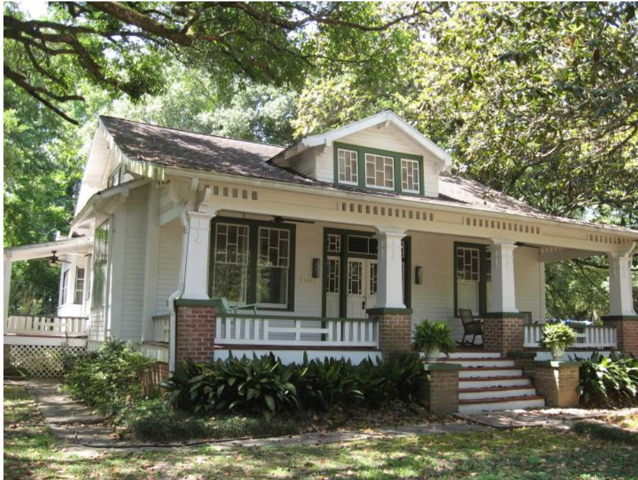
Porches help define a dwelling's style, like this Bungalow's wide porch with tapered posts on brick piers. Porch elements shall be preserved and maintained (22014 2nd Street).
