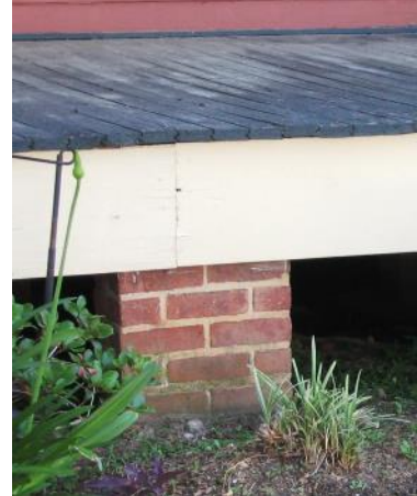
Many houses in the district have brick pier foundations that should be maintained and preserved (72104 Laurel Street).
