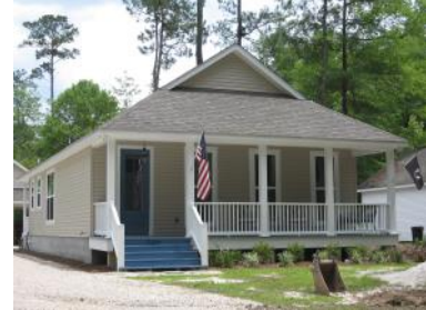
The gable-front design of this infill dwelling at 71294 St. Mary Street reflects historic house patterns in the district.
