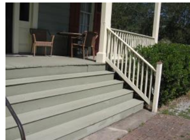
Appropriate rebuilt porch stairs and railing at 71667 Leveson Street.
