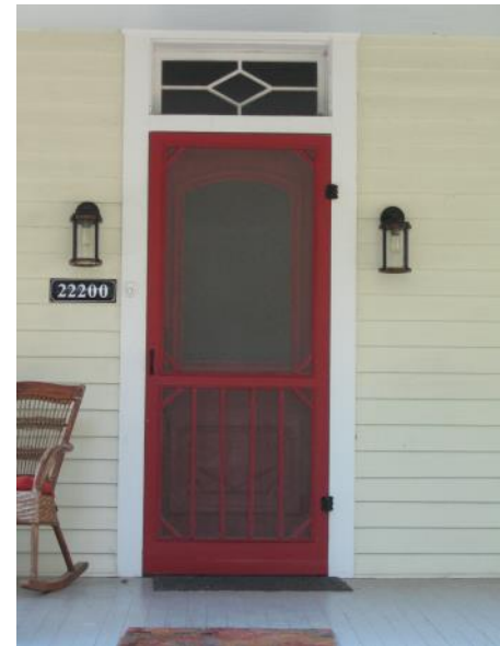
Appropriate screen door at 22200 Main Street.
