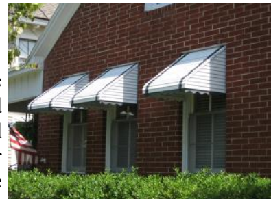
Example of appropriate metal awnings added over windows.
