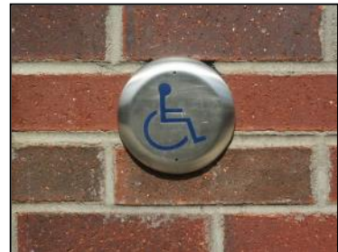
Push plates for ADA access are appropriate solutions for access into commercial buildings.
