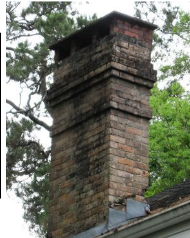
An exterior brick chimney at 22128 5th Street
