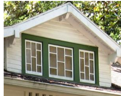
The original casement windows of this roof dormer help define the historic character of the dwelling (22014 2nd Street).
