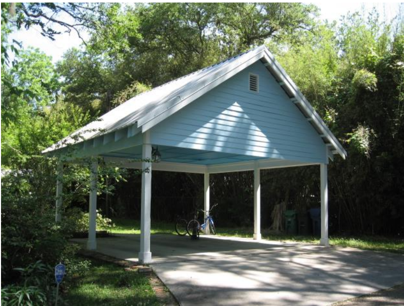
Appropriately designed carport at 71614 St. Mary Street.
