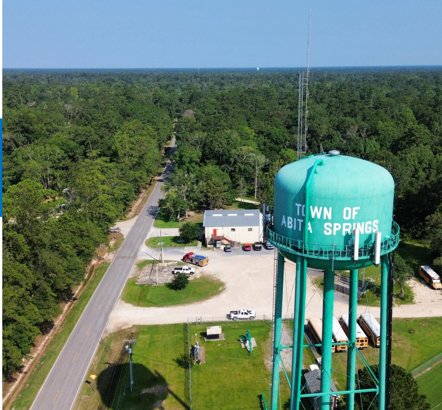
Abita Springs water tower looking northwest on LA-36
