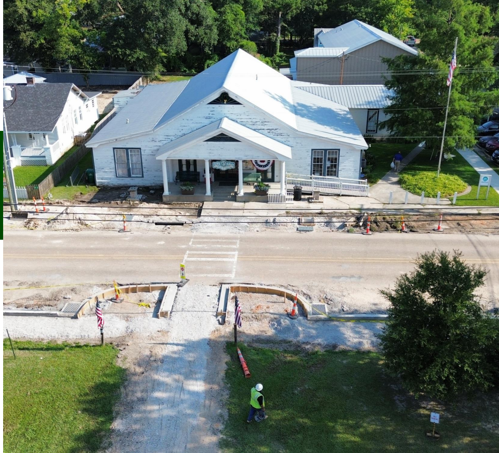
Abita Springs Town Hall during Level St. construction
